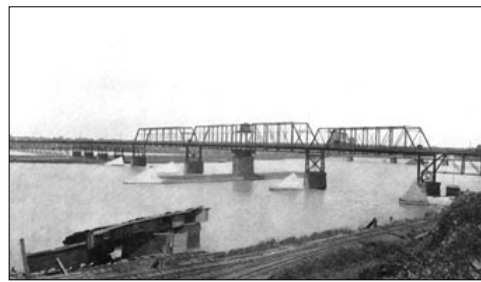
The Fasset Street Bridge.
